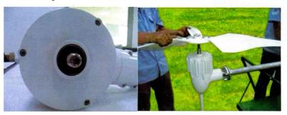
5.4.2 Tightening the hub by locking nuts and M16 spring washer, and locking up split pin.
